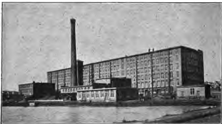
FIG. 24.—The factory shown in Fig. 23 after being equipped with an automatic stoker.
